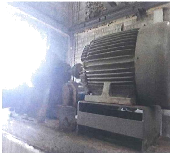
Figure 16.-Bomba de carcasa partida Reservorio EB Sur
